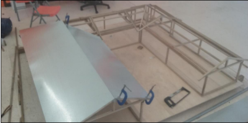
Figure 14: Installation of sheet metal.
