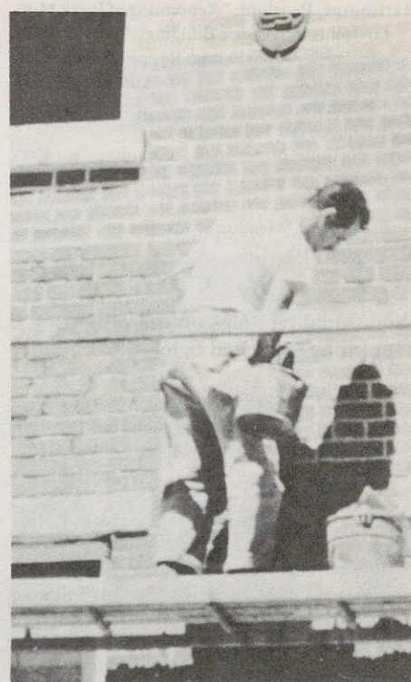
Figure 6. This photograph shows the significant visual changes which can result from improper repointing procedures. Note the increased thickness of the joints, the color variation, and the difference in the method of tooling, all noticeable even from a distance.
