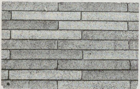
E Flush joint, one-third running bond early 20th century.
