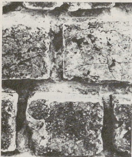
Figure 4. The damage to the edges and corners of these bricks was caused by using a power grinder in cleaning the joints. Extensive hand work is required to prevent damage to the bricks during joint preparation.
