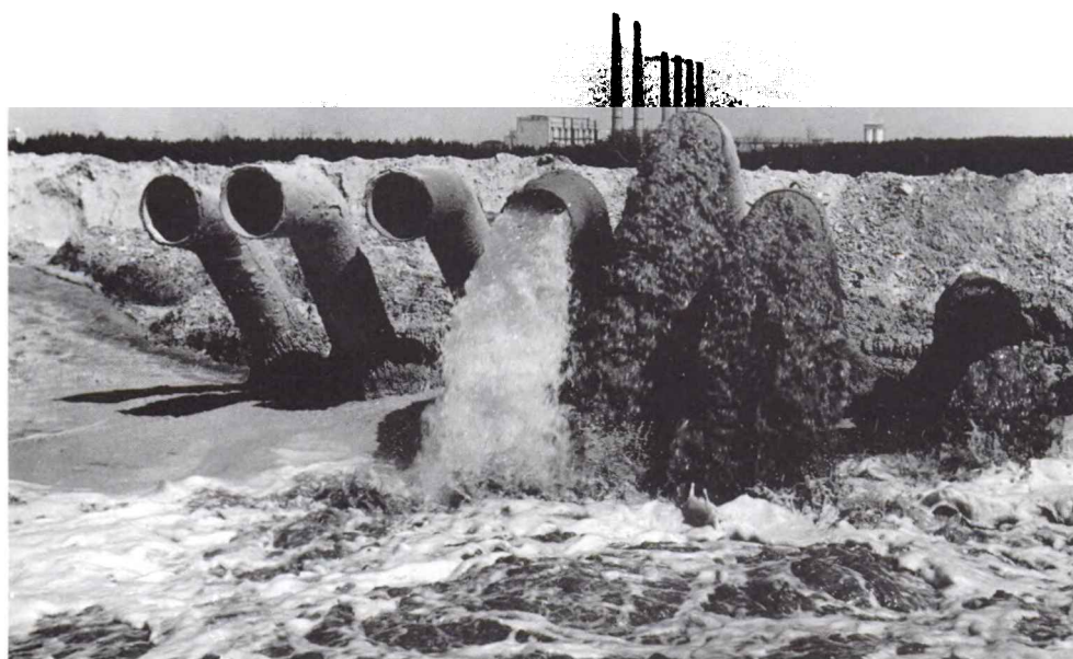
Plate 8: The Baltic power plant near Narva (north-east Estonia). Disposal of alkaline shale ash mixed with water in special reservoirs. ( Photo: Jüri Pere )
