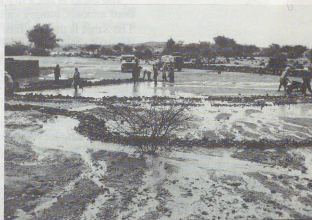
A small-scale system of dams will retain water and help rehabilitate this habitat in the Air, Niger (photo: WWF/John Newby).
