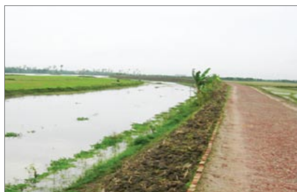
Plate 1: Road-cum-embankment constructed by local government in the Raktodaha Beel area
