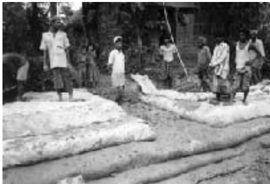
Use of geo-textile for homestead protection in Rajapur, Jamalganj
