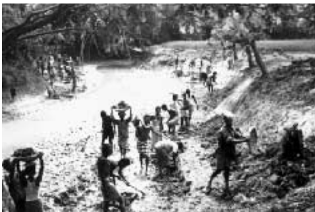
Canal re-excavation in the Boka Beel area, Trishal
