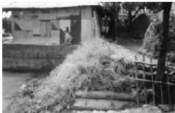
Geo-textile layers covered with vetiver grass in Rajapur
