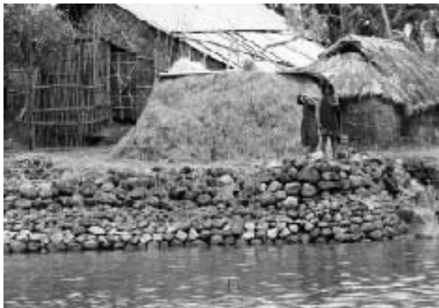
Protection measure with boulders in haor
