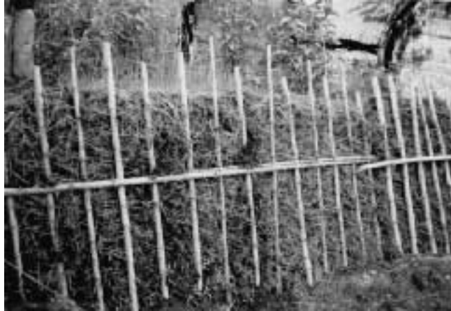
Erosion proofing with chailla in khuti bundh
