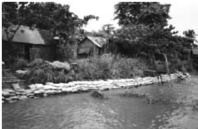
Homestead protection in haor using sand-bags
