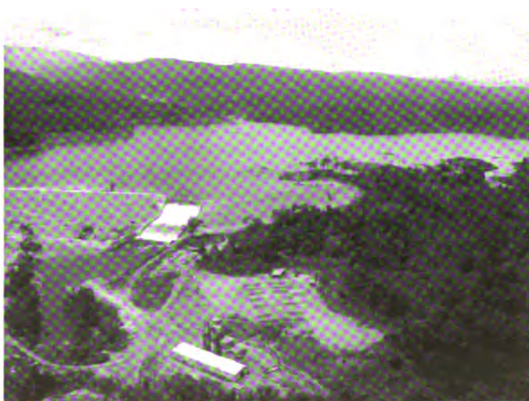
Nam Leuk hydro-power project, Bolikhamxai Province
