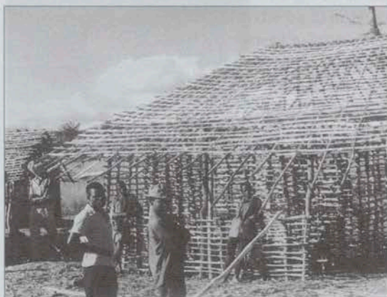
Local knowledge and community involvement in the construction of a check-point in Puíla, in the Sanga District, in Niassa Province.
